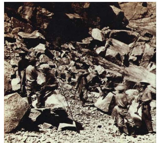
Labors near the opening of Summit Tunnel, Central Pacific Railroad
