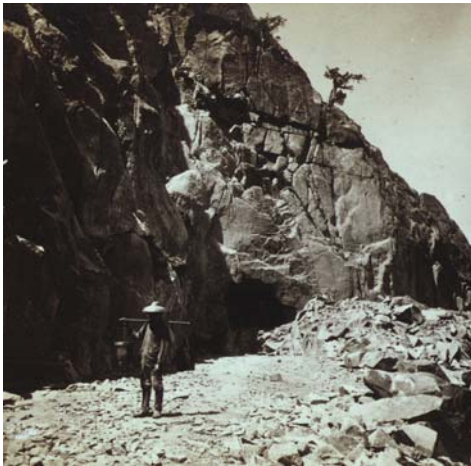
Heading of east portal Tunnel No. 8, Central Pacific Railroad
