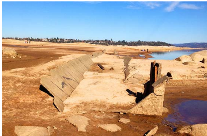
Keystone arch aqueduct of the Negro Hill Ditch west of Salmon Fall on the north side of the South Fork of the American River
