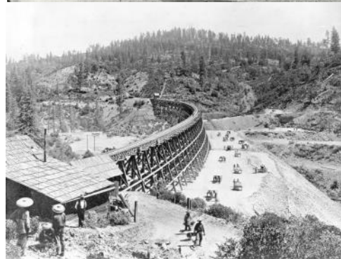
Top: Central Pacific Railroad Bottom: Chinese workers at a trestle, viewed from an overlook
