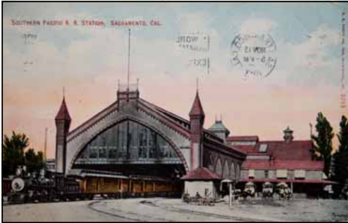
Above: This postcard of the former Southern Pacific Railway Station on G Street is postmarked November 13, 1913. The building was torn down later. Color image © T. Myers Photography
