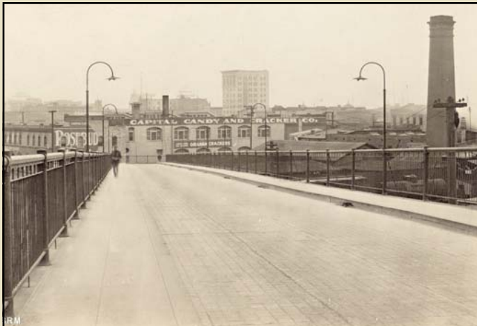
I Street Bridge - Jiboom St. exit ramp, 1912. California State Railroad Museum
