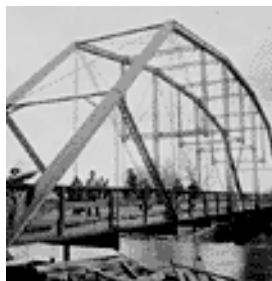
Meiss Road Bridge, 1894. CSRM Library
