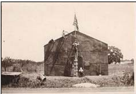
Local residents restoring the Sutter Hock Farm facade ca. 1927. Photo E. von Geldern, via Wikipedia
