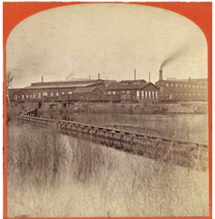
C. P. R. R., Shops, Sacramento, Cal., J.J. Reilly, Marysville, Calif., [187-?]. View looks northwest across Sutter Lake. At left are Hammer shop and Rolling Mill. Power House Tower is at right rear.
