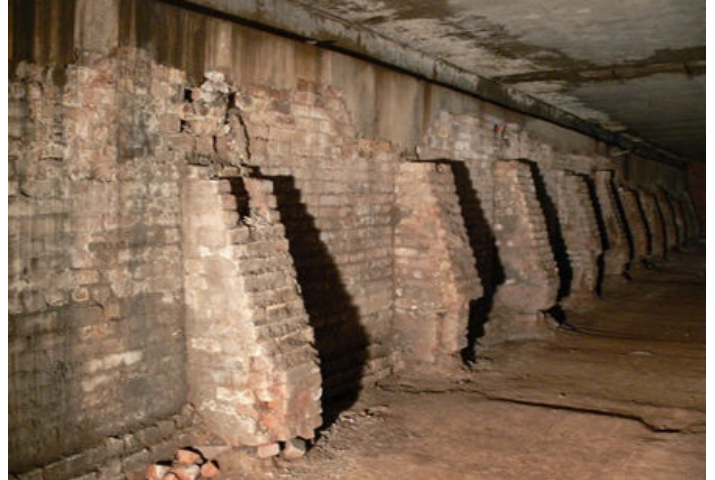
Exposed footings revealed under raised Old Sacramento Center for Sacramento History
